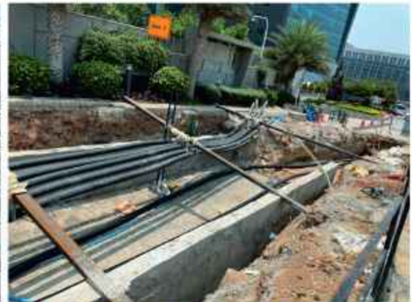
220 kV EHV Cable Laying for 400 kV Raidurgam Sub-Station
